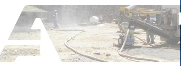
The Airplaco C-10SL gunite machine provides maximum performance and efficiency due to its heavy-duty design and powerful output. The C-10SL dry-mix gunite machine features a premium-life feed system, molded discharge liner and exhaust suppression chamber. A tilt-hopper provides easy access for cleaning and setup. All units include air line regulating valves, choice of high or medium-production feed system and hopper assembly. An air compressor is required to power the C-10SL shotcrete machine.
