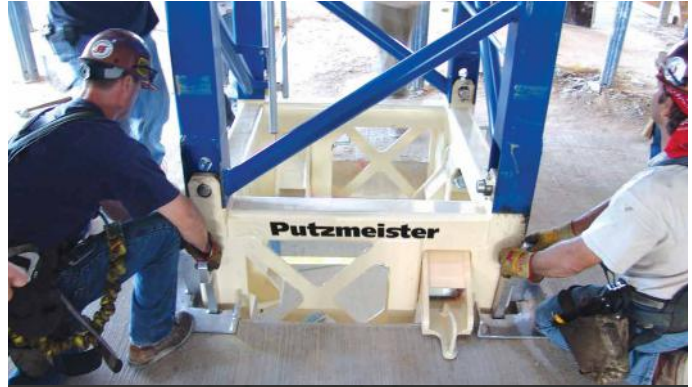
SIMPLE BRACING WITH VERTICAL SUPPORT
