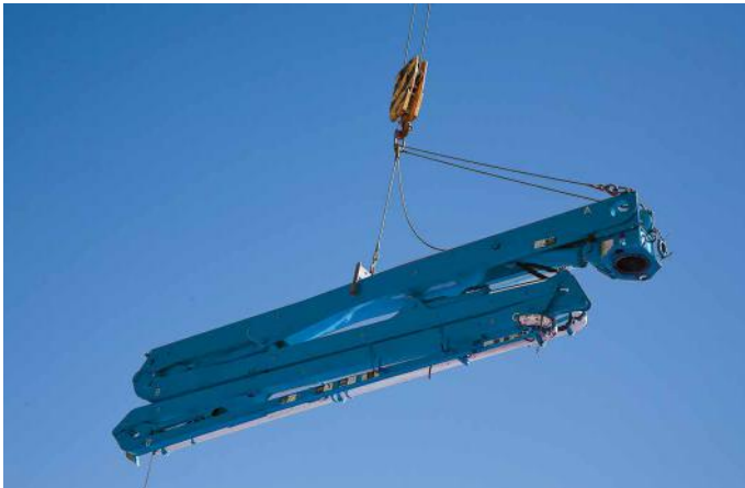
STEP 3 – Fly boom from truck to tower
