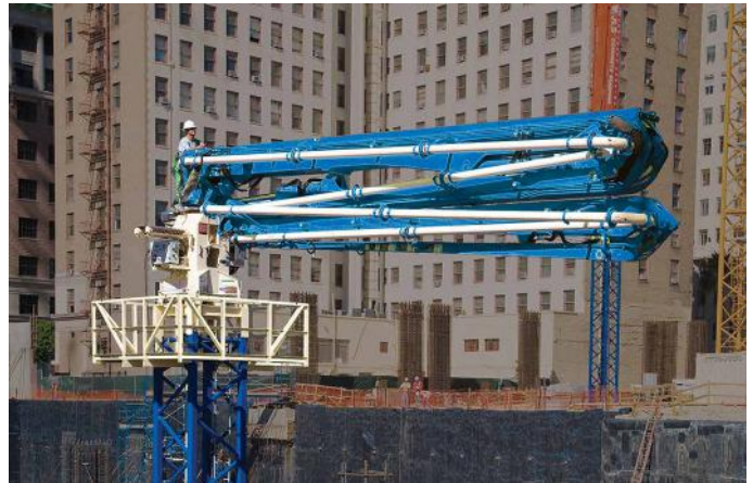
STEP 4 – Position, pin and pump
